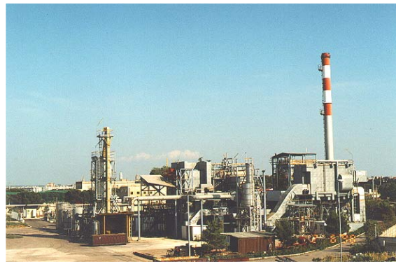
Figure 2: 50 MWt boiler overview.
